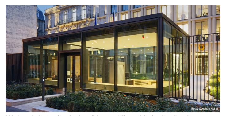
A fully-glazed, cube-shaped guardhouse for a German Embassy abroad with a security facade made from box profiles and an aluminium add-on construction, which is able to bear the 2+ tonne weight of the  $4.6 \times 3.2 \, \text{m}$  individual security glazing with ease.
