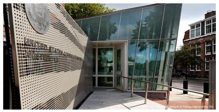
Generous glazing of the guardhouse for an American property with a sloping double facade and roof construction. All of the components were security-tested in advance in accordance with specifications of the US Department of State.
