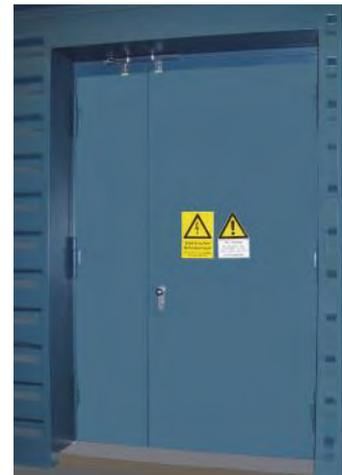
Double steel door, explosion resistant, with closing sequence control for a pumped storage hydro power plant.
