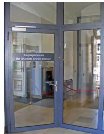
Entrance into the interlocking door system for security control.
