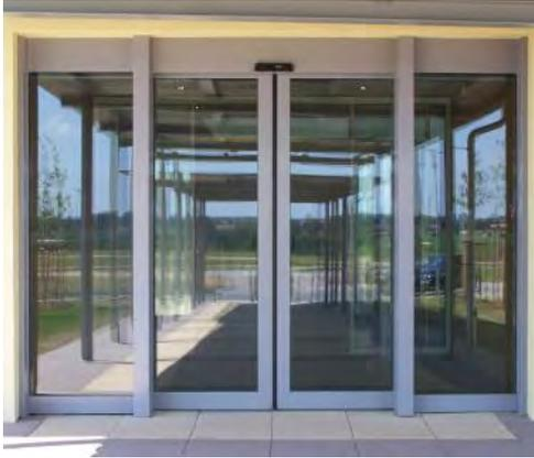
Blast resistant aluminium sliding door with side panels.
