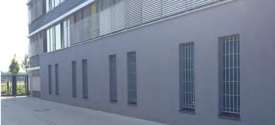
The production of forced entry and break out resistant **OXIR®**-grilles is subject to continuous external monitoring with regular control by the VdS, Cologne.
