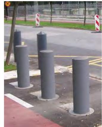
Combined automatic retractable and fixed bollards.
