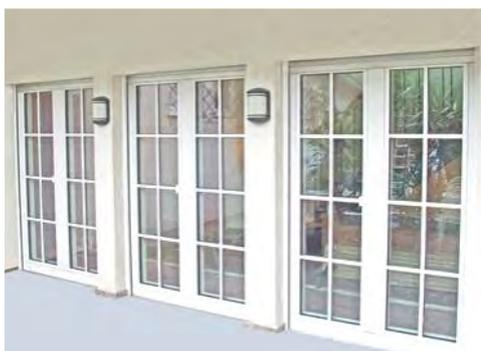
**SECURON<sup>®</sup>** is available as single or multiple window elements, with tilt and tilt-turn hardware. **SECURON<sup>®</sup>** is also available as double sash patio door, wing sizes up to 1.60 x 2.40 m.
