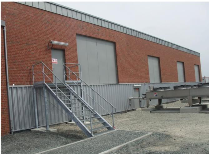
Double sliding gate, roller rail on the top.
