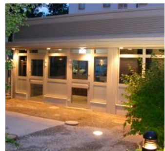
Guard houses & security entrances.
